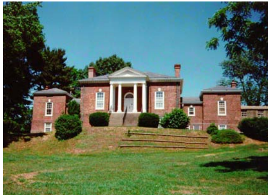
Elkins Building, Bucks County Historical Society (82-22)
